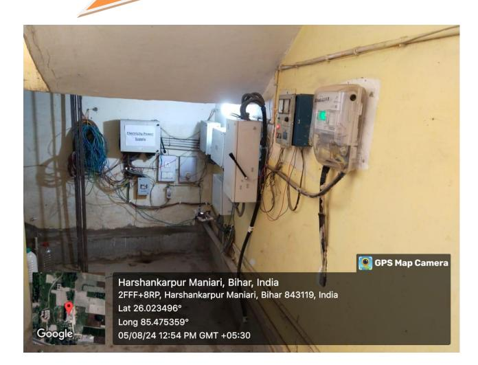
This is Electricity Borad installed in College for the purpose of Control alternate source of energy.
